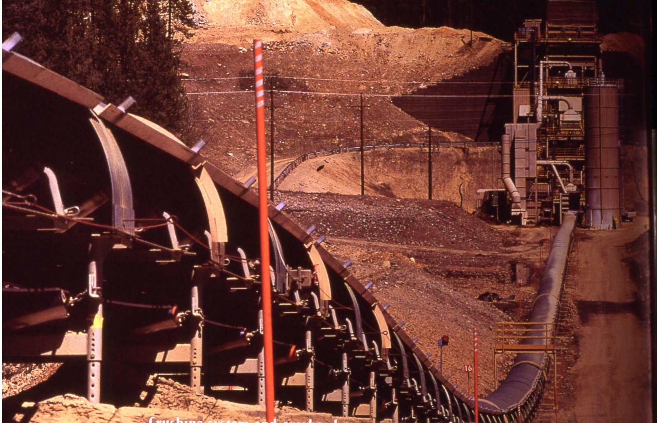
Crushing system at level 1
