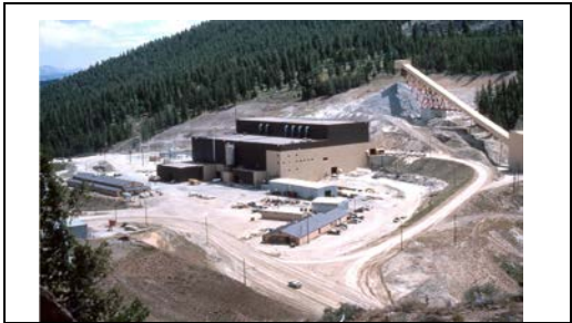
Thompson Creek Moly, Mill and concentrator, with end of conveyer.
