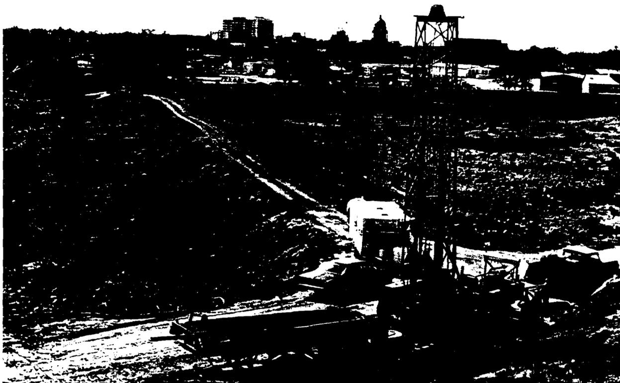
**Figure 2.** Well BHW-1 of Boise space heating demonstration project. Well flowed 194 gpm with outlet temperature of 167°F. Some of state buildings including capitol to be heated by this project visible in distance.
