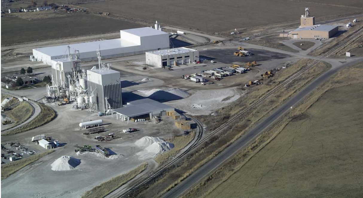
Figure 7: Hess Pumice and Owens-Corning's new Cultured Stone plant in Malad is large white building. Idaho Minerals' new perlite expander plant is in upper right.
