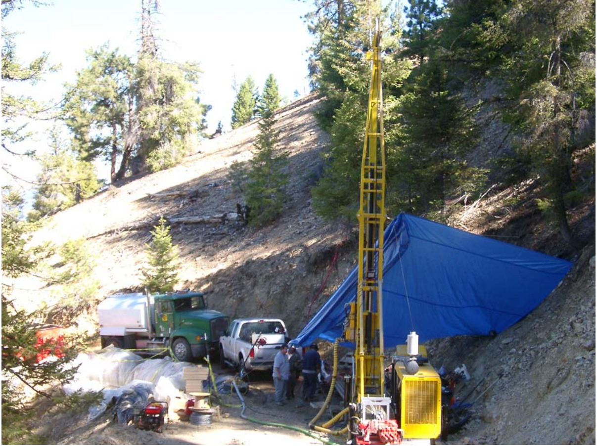
Figure 4. Drilling Hole C07-31 at the Cumo Property, Boise County, Idaho.
