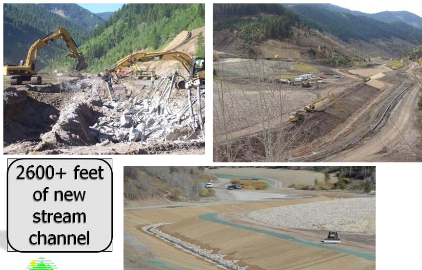
Figure 8. Agrium/Nuwest's Georgetown Canyon Remediation project.
