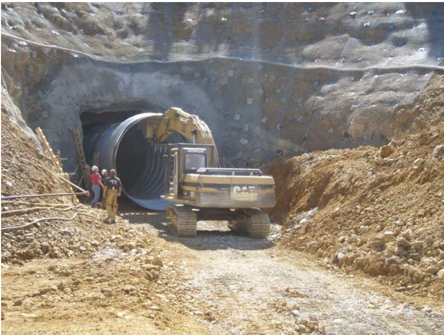
Figure 14. Portal of the Countess Decline, Crescent mine.
