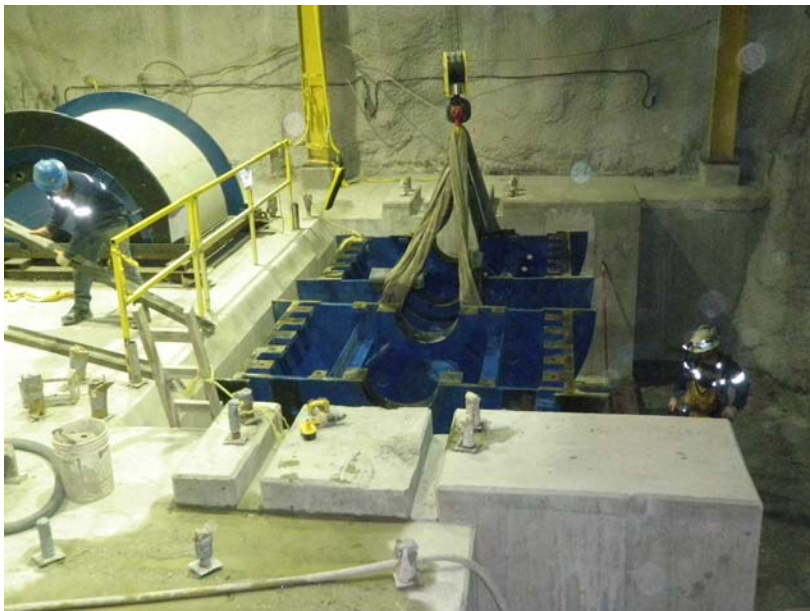
Figure 4. Installing hoist drum halves, # 4 shaft, Lucky Friday mine.
